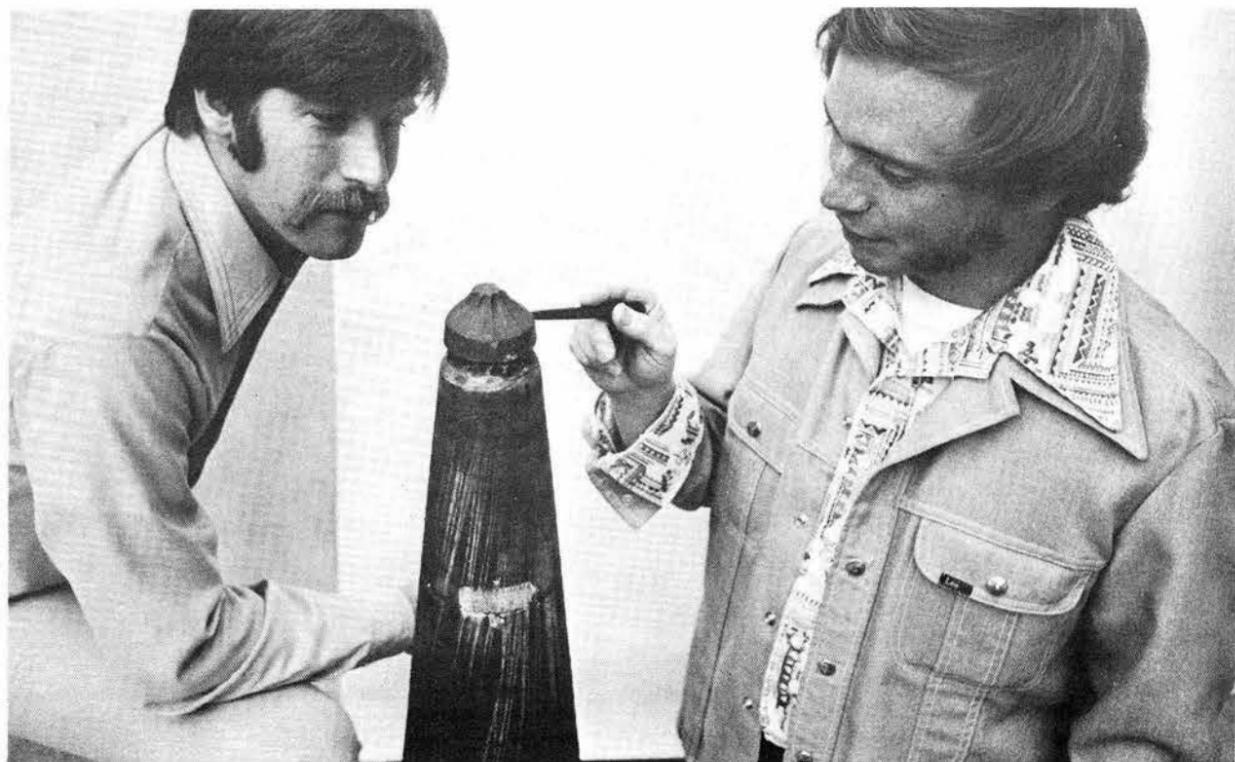
RECOVERED NOSETIP, no longer hemispherical, is focus of Ralph Clark's and Ed English's attention. Streaks are aluminum melted by heat generated at the tip.
