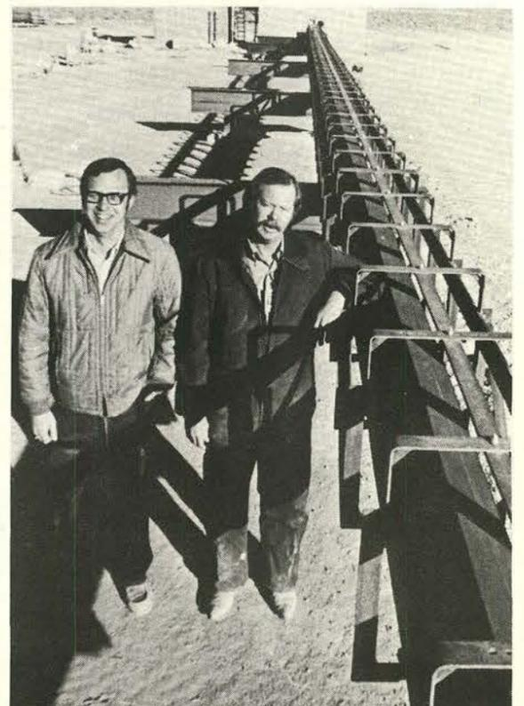
ROCKET SLED track at TTR used for the tornado safety studies is constructed from steel I-beams with welded safety cage. At left is project leader Al Stephenson with Jack Windsor (both 9473).
