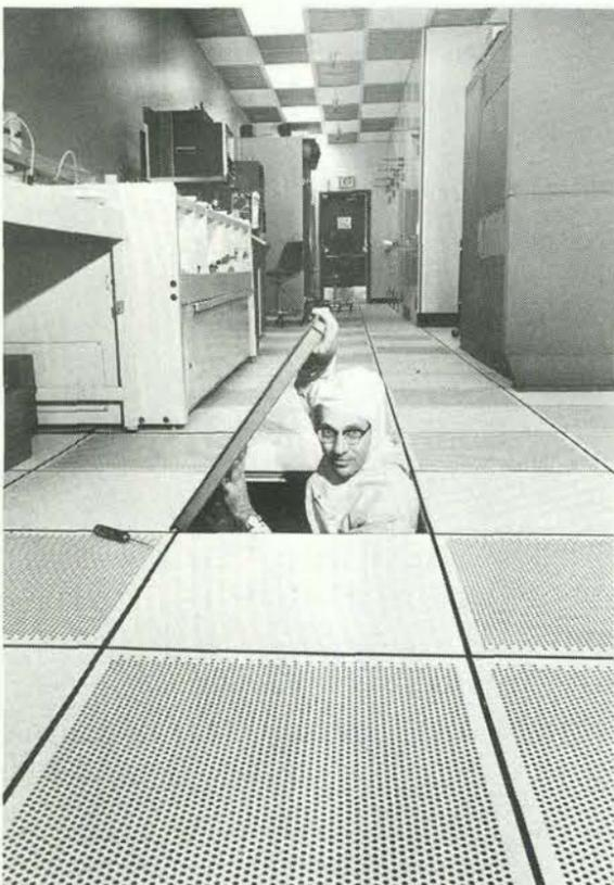
CHARLIE BARNES (2141) solves one last water leak under the floor of new clean room area in Bldg. 870. Filtered air flows constantly from ceiling to floor to provide super clean environment for the fabrication of IC devices.
