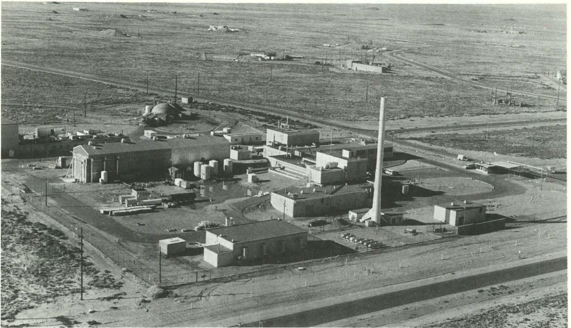
SITUATED on the mesa next to Area III, the Labs' reactor area (Area V) consists of a complex of reactors designed to support the research and development activities of Sandia. Annular Core Pulse Reactor (ACPR) plays key role in breeder reactor safety program described below.
