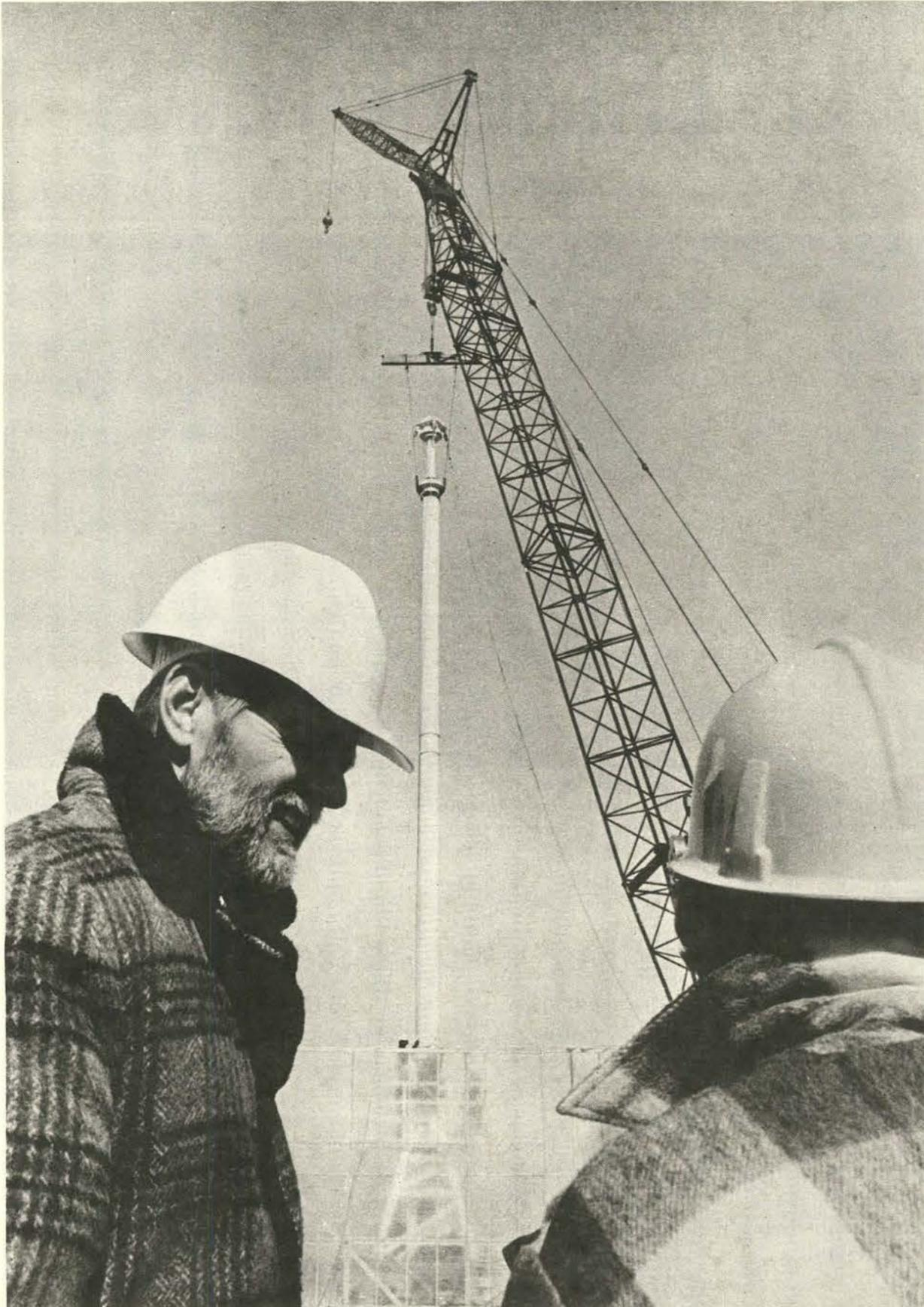
NEW WIND TURBINE SHAFT, is emplaced on a 5.5 m base east of Area I. With the anemometer tower added later, total height is 33.5 m. The revolving shaft will eventually support three experimental blades (arranged to form a 17 m diameter sphere) and drive a generator. Here Bob Grover and Carl Longfellow (both 5715) debate the delights of riding a crane-lifted cage to bolt on the anemometer tower. (Both lost out to Ralph Rusk, also 5715.)
