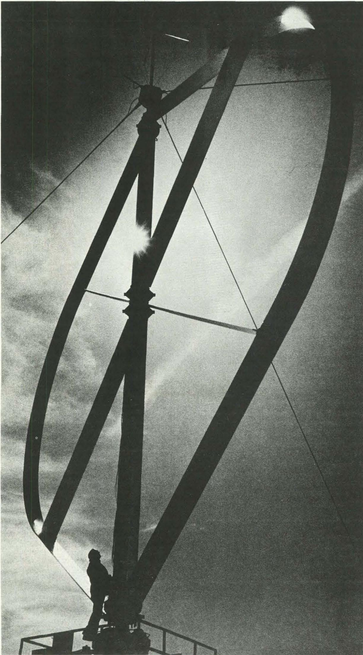
INITIAL TESTING of Sandia's new vertical axis wind turbine is underway at its East Mesa site. The turbine, as tall as a seven story building, carries egg-beater-like blades 17 metres in diameter. Winds in excess of 10 mph enable the turbine to produce power. Emil Kadlec (5715), project engineer, expects the initial testing to continue for several weeks. A third blade will be added to the turbine later this year.
