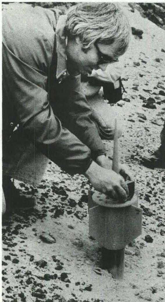
MARS-man Eric Reece (1327) examines prototype penetrator following test drop in Mars-like soil.
