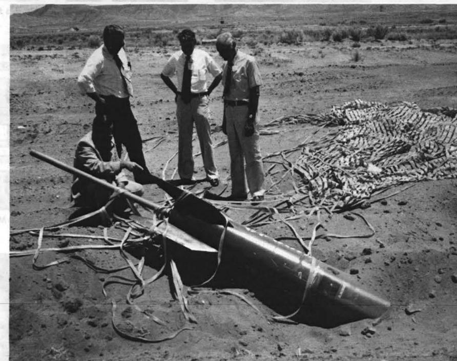
KEVLAR PARACHUTE TEST on the rocket sled track facility in Area III was witnessed recently by the Army's Maj. Gen. Milton Key, Deputy Assistant to the Secretary of Defense for Atomic Energy, second from right. The new parachute material, stronger than nylon with less bulk, allows a greater diameter parachute to be used on the B61 laydown weapon. From left are John Duncan (4312), test engineer; Bob Puerifoy (4300); Maj. Gen. Key; and President Sparks.
