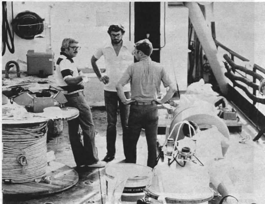
ON BOARD the Coast Guard ship "White Pine" in the Gulf of Mexico are Eric Reece (1327), Lou Feltz (1324) and Dave Ryerson (1327). In right foreground is the Sandia Acoustic Telemetry System which successfully transmitted and received high data rate signals through sea water.
