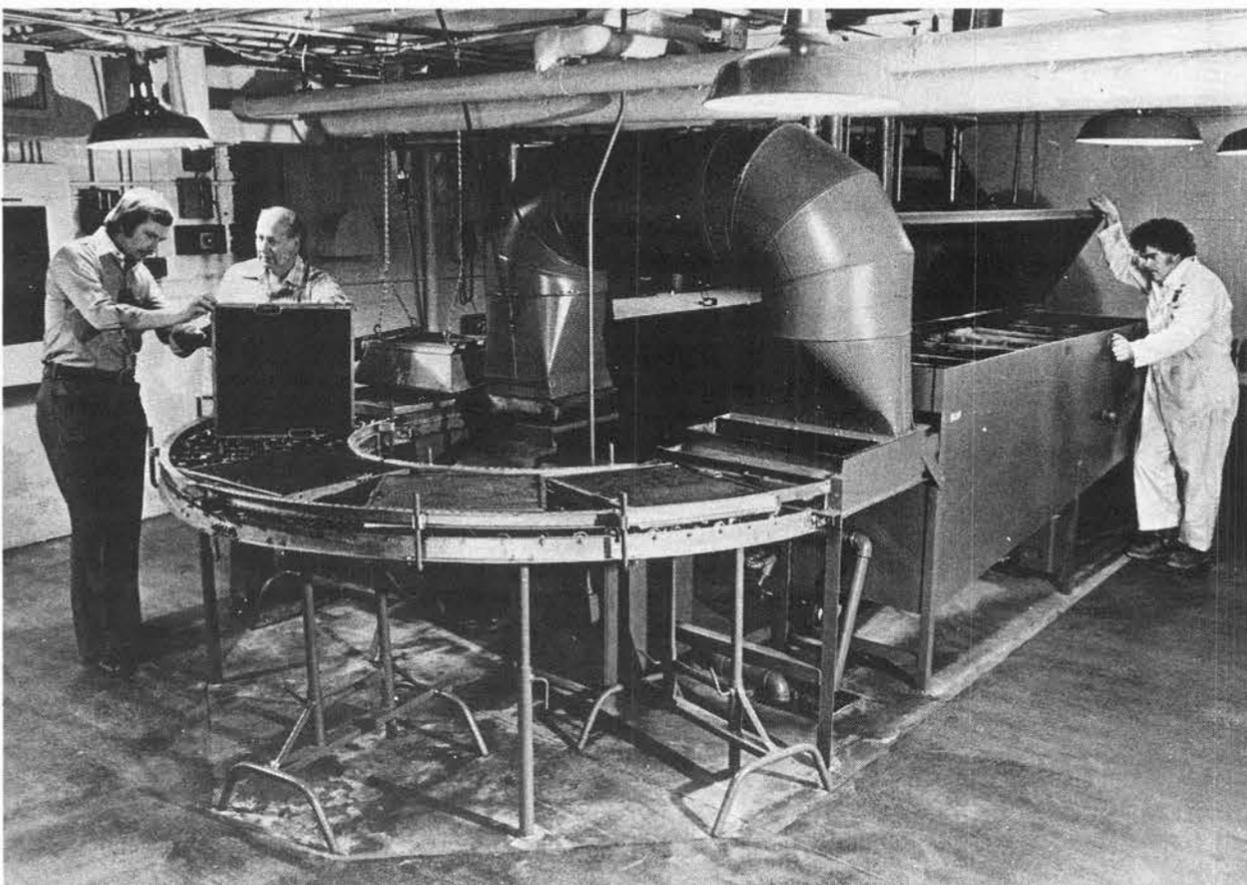
PLANT ENGINEERING's Al Dickinson (9743), at left, is chiefly responsible for the design of the Lab's filter cleaning plant. Some four to five thousand air filters are washed, dried, and oiled each month in the automated plant. The filters are used to clean intake air throughout the Labs. Bud Hall (3422) is shown with Al, while operator Abedon Ortiz (also 3422) is at right.
