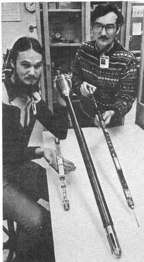
**FOR GEOTHERMAL WELLS**—New logging instrument which measures downhole temperatures up to 300°C is displayed by Kyle White and Dave Palmer (both 2151). Two versions of the electronics have been tested—hybrid thick film technology (which Kyle holds) and a system using printed circuit boards.
