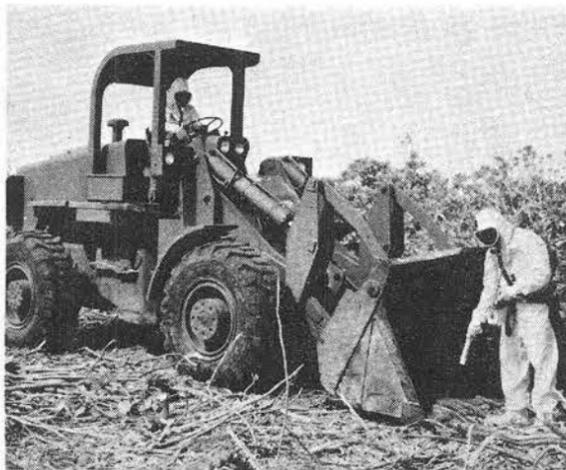
PLUTONIUM in the top soil is scraped up by bulldozers, mixed with concrete and dumped into a restricted area. Few areas remain where anti-C suits are needed.
