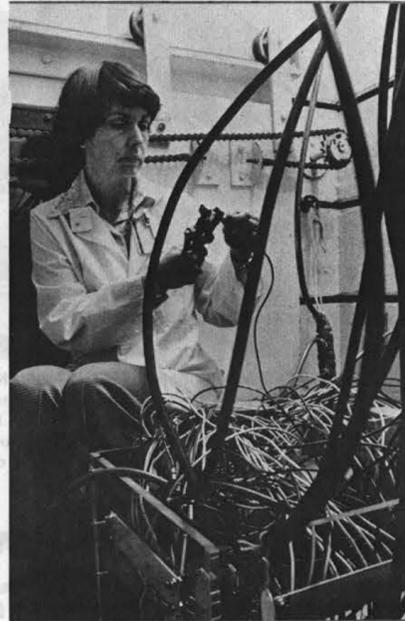
BARBARA STEARNS (5432 - ESA Trainee) works on test setup used to measure effects of radiation on nuclear reactor cabling.
