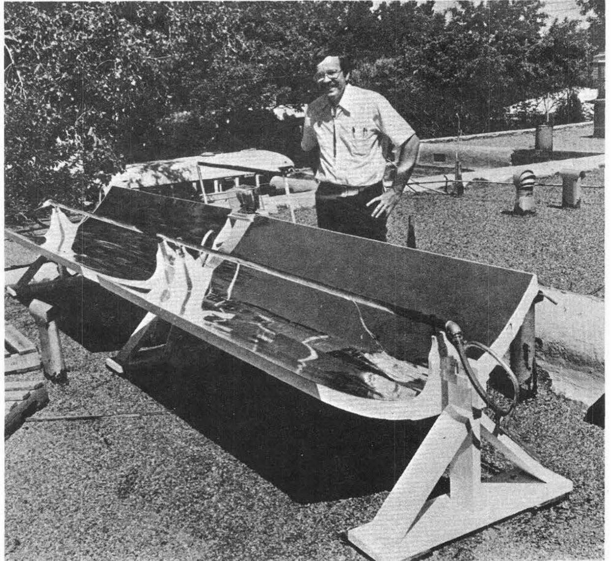
UP TO THE SUN. Bob Stromberg (5714) uses solar energy to heat hot water for his home. Sensor he designed and built tracks the sun and keeps rooftop parabolic collector troughs properly oriented. Entire system was built in about five months (nights and weekends), mostly from surplus materials.
