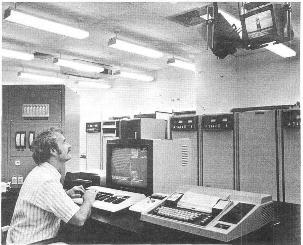
DAVE DARSEY (1521) operates the master control system at the Solar Thermal Test Facility (Power Tower). Automated controls use a network of minicomputers to integrate operations and data acquisition.
