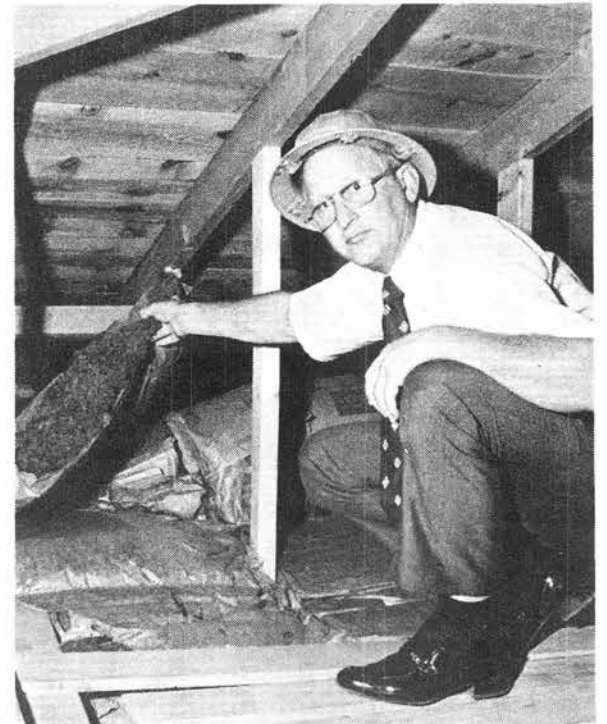
DAVE WEINGARTEN (2153) added six inches of insulation in his attic to bring the total to 12 inches. He realized significant savings in his fuel bill.
