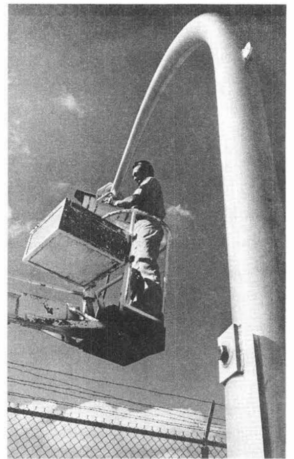
ORVILLE HOWARD (1733) adjusts aim of TV camera over a security fence. Special camera support standard was also developed by Sandia for the Air Force as part of new CCTV security system.
