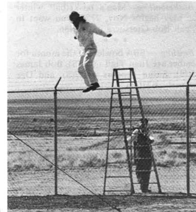
BILL INGRAM (2454) demonstrates stepladder launch over fence. No-touch technique means that fence sensors would not be activated by this type of intrusion.
