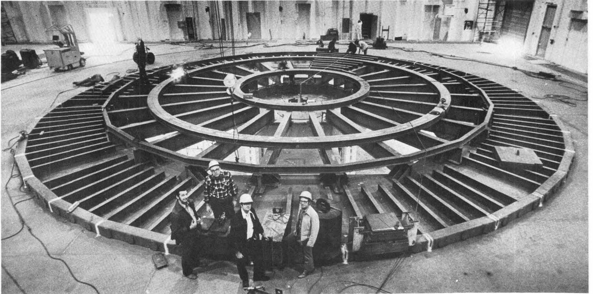
STEEL SUPPORT STRUCTURE for Sandia's EBFA-I (Electron Beam Fusion Accelerator) is shaping up in the new facility building south of Area I. Components of EBFA-I are being fabricated in machine shops throughout the state. Accelerator assembly should be complete and the experiment operational in June 1980. In the meantime, construction of a new office and laboratory building is nearing completion; occupancy by the staff of Fusion Research Department 4240 and Pulsed Power Systems
