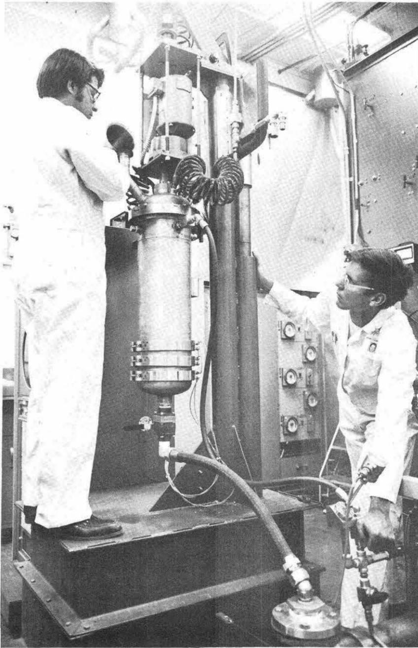
JIM LYONS & DAVE HAWN (both 4371) are shown with bench-scale reactor which is used to study how coal liquefaction process can be made more efficient. They are adding a coal slurry to the reactor preheater in experiment to identify what happens in early stages of coal liquefaction.
