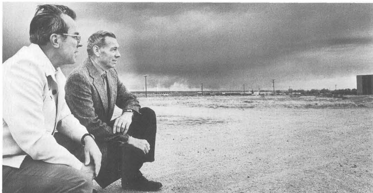
BOB NEEL (4731) and HUGH LEENHOUTS (DOE), members of AARC's Building Corporation, survey building site for two "group homes" specifically designed for residents confined to wheelchairs. Construction will begin in June.
