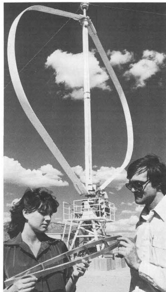
NEW BLADES have increased the efficiency and electrical output of Sandia's vertical axis wind turbine. Sheila Guynes and Bill Sullivan (both 4715) examine a cross section of the new blade. The new blades are fabricated by an economical extrusion process.
