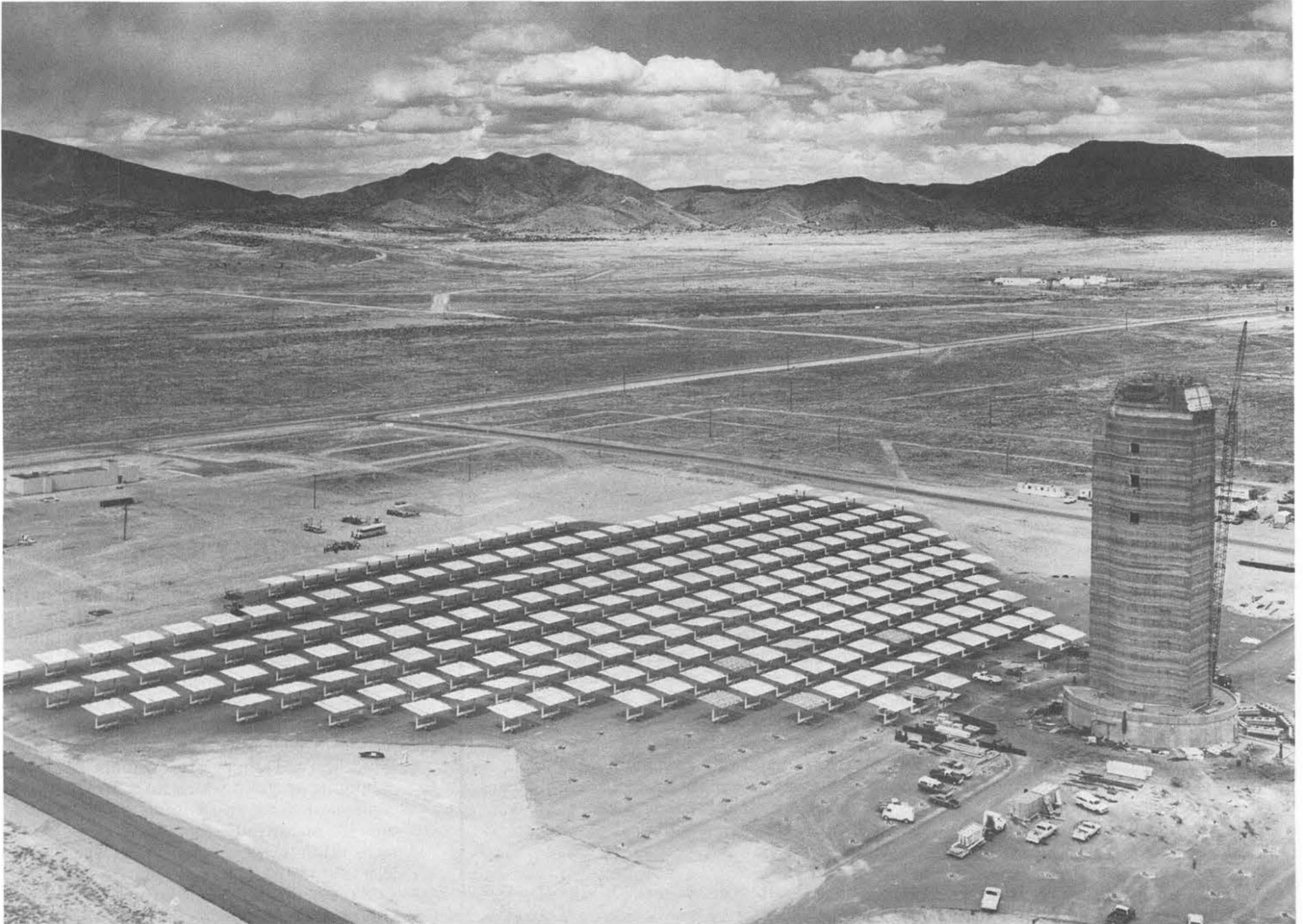
AERIAL view of Sandia's Central Receiver Test Facility — the Power Tower — was taken shortly before facility was completed. Experimental boilers have since been installed and testing is underway. An unusual night-time experiment was recently completed here, using the array of
