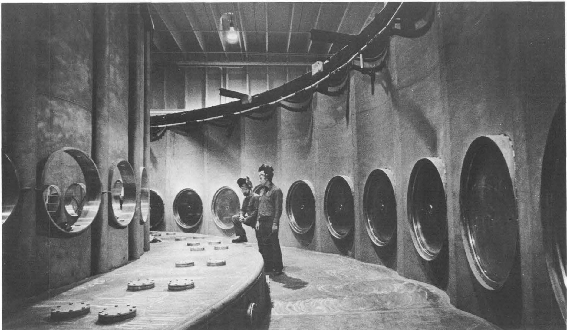
**PARTICLE BEAM FUSION ACCELERATOR**—Major construction work on this facility in Area IV has been completed, and it is expected to be in operation by next fall. It will have a dual capability: to accelerate electrons, producing intense bursts of x-rays to simulate nuclear weapons effects; and the
