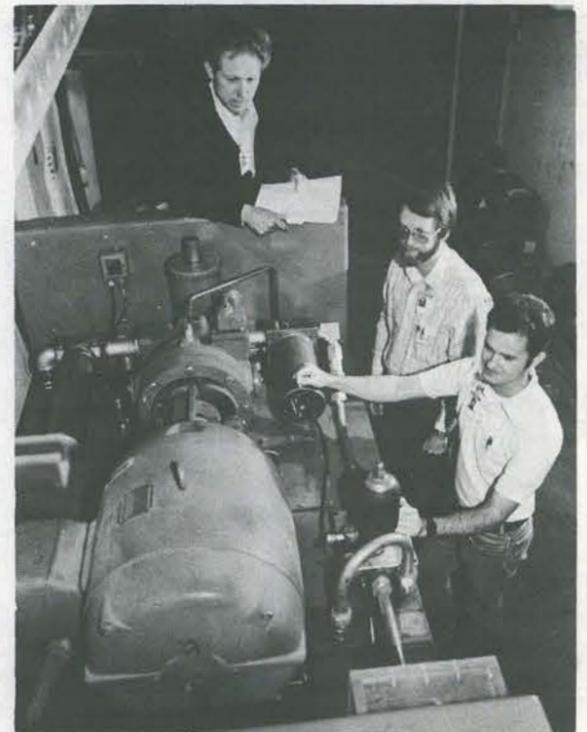
DISCUSS ENERGY SAVINGS—Earl Gruer (3652), Jim Van Den Avyle and Bob Cross (both 5835) plan exchanging this pump and motor installation in the basement of Bldg. 805, which powers 24 hour per day long term mechanical stress tests, for a smaller unit requiring less electricity to operate. The exchange will save a significant amount of energy and money.
