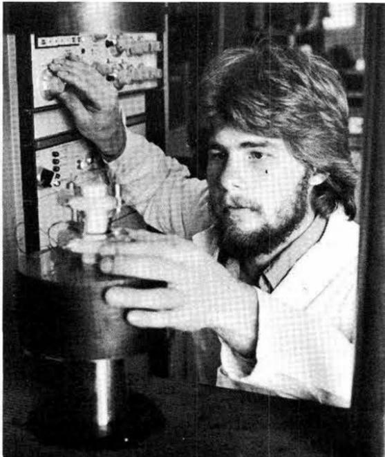
JERRY O'BRIEN adjusts rock sample for a uniaxial compression test to measure stress/strain response.
