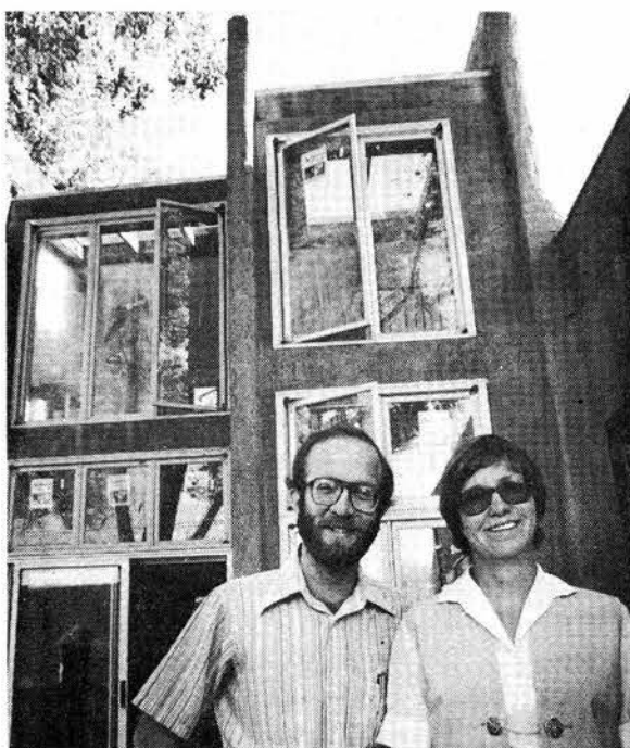
GLASS WALL on south side of two-story addition to the home of Harold and Chris (2614) Morgan is part of a passive solar space heating system.
