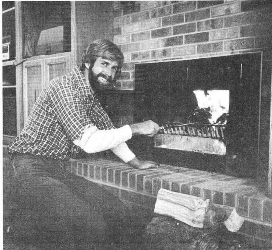
DAVE BAGLEY (DOE) stokes his wood-burning custom fireplace furnace. Note two small muffin fans at bottom corners of unit. They circulate inside air around the firebox and back into the living area to heat 1500 sq. ft. of space. With glass door closed, the flame pulls outside air through the ash removal trap and vents it out the chimney.
