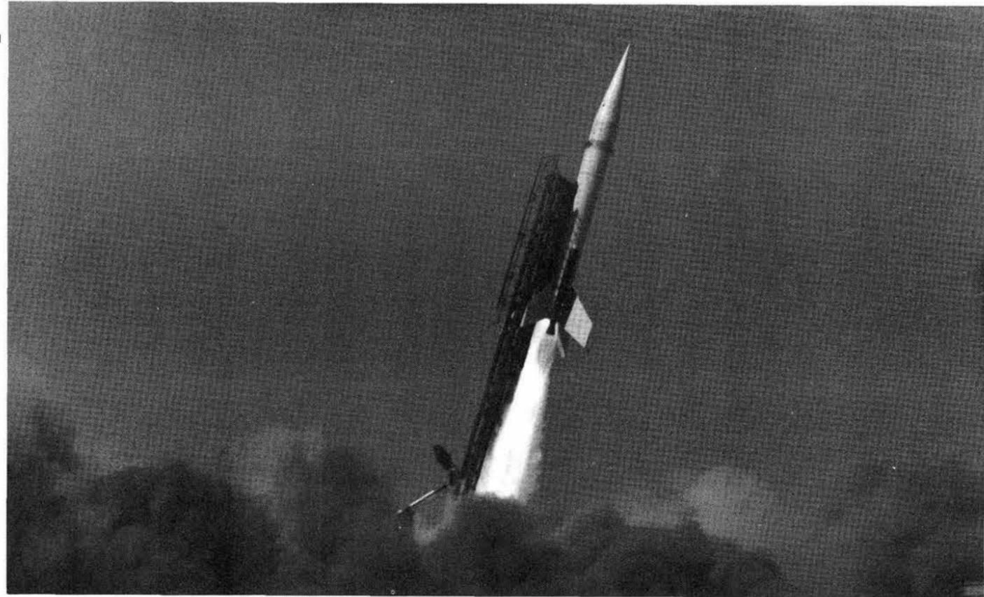
SWERVE II, a highly maneuverable, inertially guided RV developed in Dept. 5620, was successfully flight tested in a STRYPI VIII-R rocket last September. Here test engineers from Org. 1500 ready vehicle for launch at Pacific Missile Range Facility in Hawaii. Launch photo was taken by Gene Moore (3153).
