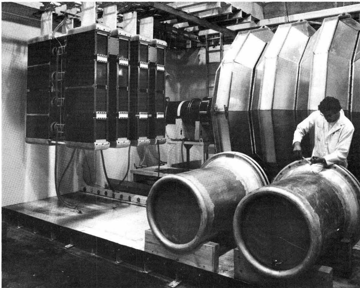
**UNDER the Labs' pulsed energy program, construction was high-current, radial-pulse line, linear accelerator in this completed and initial operations started with the first country. (4250)**
