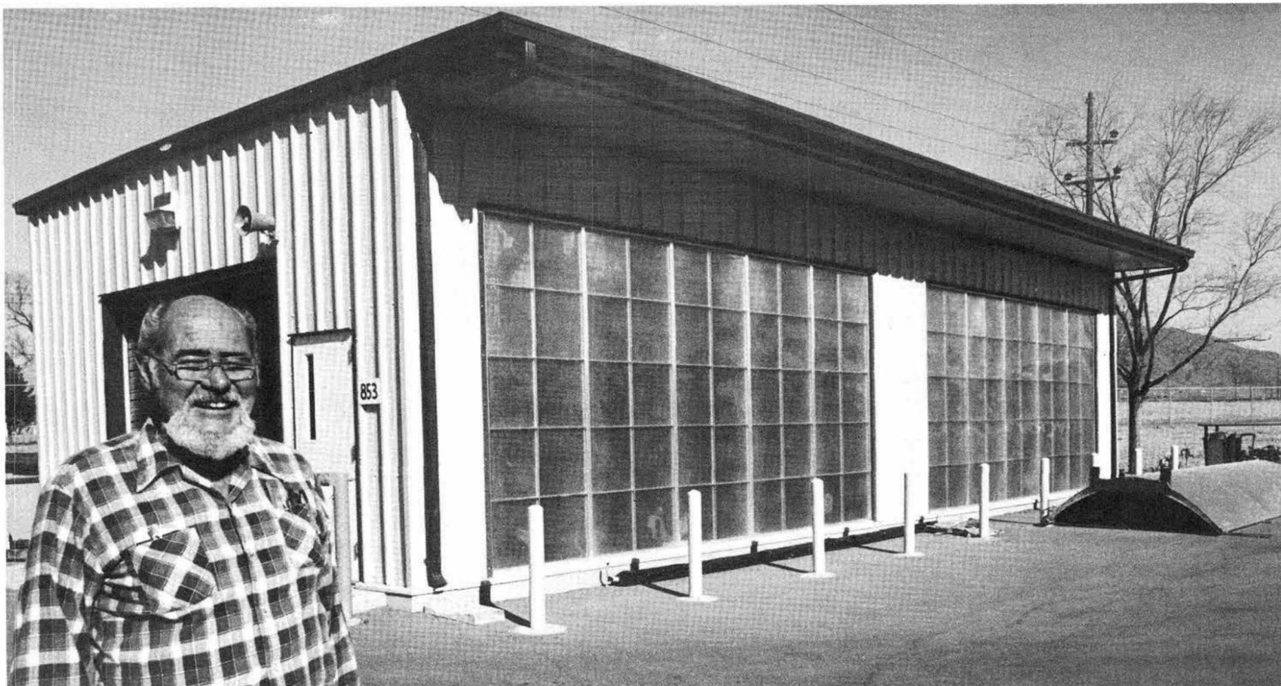
VERY COMFORTABLE is the way Larry Rodke (EG&G/4721) describes the interior of a solar-heated assembly building in the Photovoltaics Advanced Systems Test Facility. Larry works in the building every day—last winter he needed auxiliary heat only one morning following a four-day period of cloudiness and cold temperatures. The translucent south wall admits winter sunlight to heat 26 water-filled black fiberglass cylinders just inside the wall.
