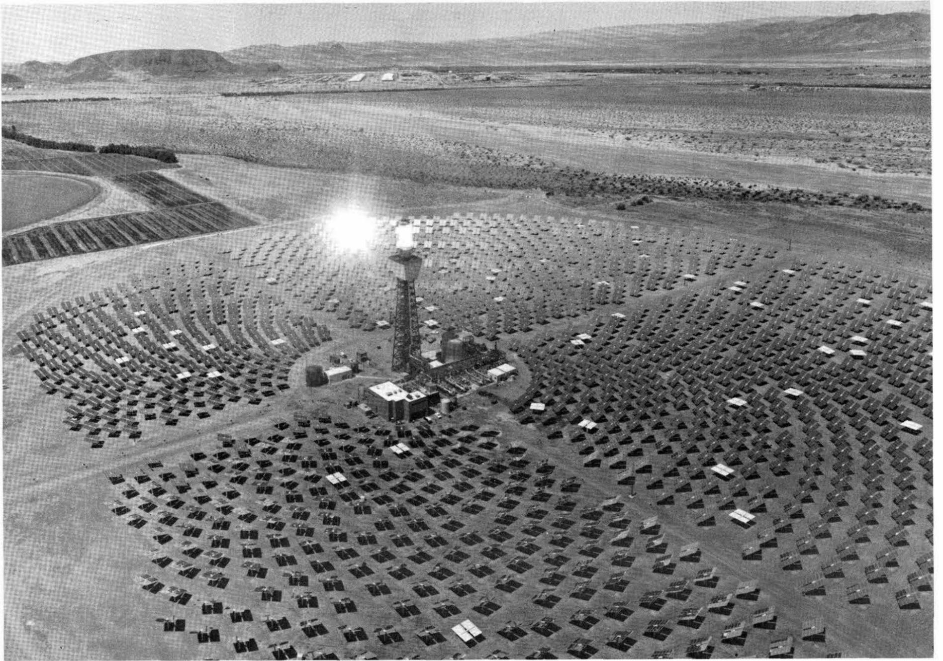
FIRST ELECTRIC POWER—A field of giant heliostats reflects the sun's rays to Solar One's boiler/receiver atop a 300-ft. tower to produce super-heated steam
