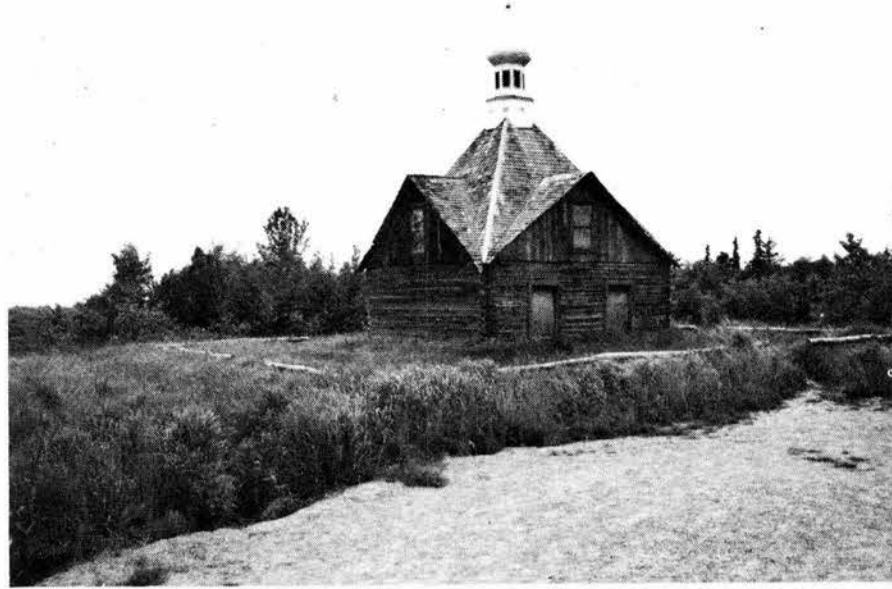
OLD Russian chapel being restored at Kenai.
