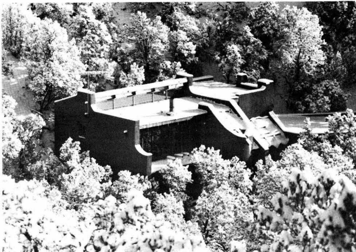
BOB HARNAR (7417) took this picture of his passive solar adobe house in the Sandias after a snowfall last winter. A large clerestory and solar greenhouse are features of the south-facing facade. Note horseshoe-shaped entryway, which holds a solar collector for the hot water system on the roof. Garage workshop extends to the right behind the trees.
