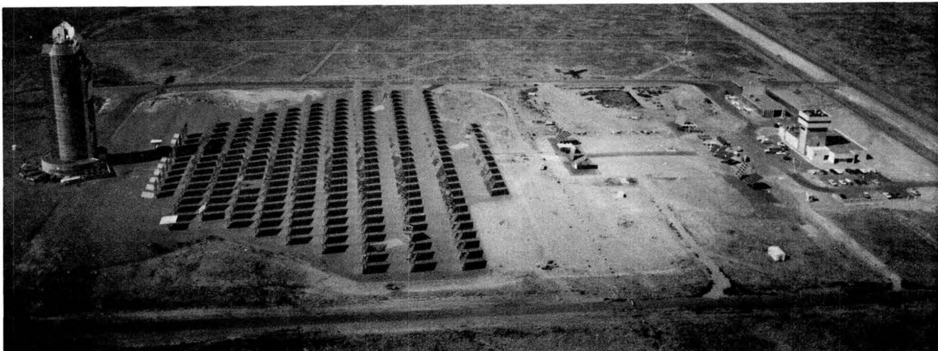
CENTRAL RECEIVER TEST FACILITY was the site of a Molten Salt Electric Experiment, the first US system to use molten salt rather than water to transfer
