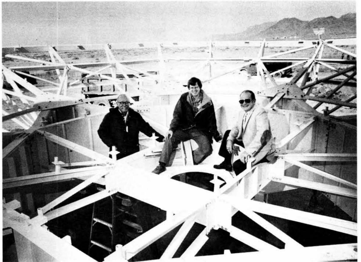
SHAPING UP NOW at a site adjacent to Sandia's Power Tower is the first of eight large parabolic dish reflectors that will comprise a new Distributed Receiver Test Facility. From left are Hal Baxter (6222), in charge of construction; Chris Cameron (6222), DRTF project leader; and Bob Hunke (6227), parabolic dish project leader. The dish, a test bed concentrator, will be 36 feet in diameter, mounted on a 45-foot-tall pedestal.
