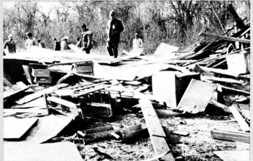
high explosive was detonated. Some damage resulted (left corner) when a desk and other office furniture smashed through the wall. The structure was repaired, and an identical charge was exploded. Results are illustrated in photo at right. The foam reduced blast effects tenfold and trapped more than 90 percent of particulate matter.
