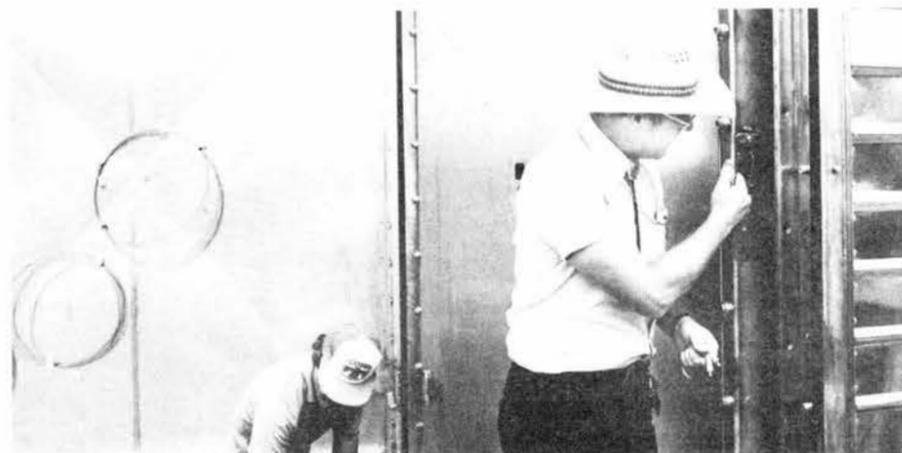
LEAK TEST PORT on inner door seal is checked by TRUPACT Project Leader Vern Romesberg (6322). Outer door behind him has same construction as the outer steel box — a steel tube framework covered on the outer surface with stainless steel sheet. Inside the frame, layers of Kevlar (like that used in bullet-proof vests) and stainless steel serve as puncture shields.
