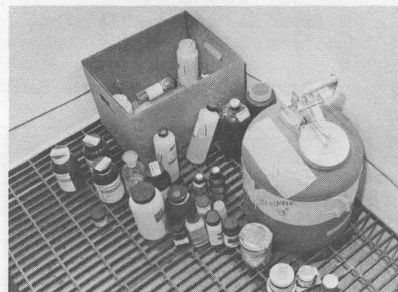
CHEMICAL WASTES, separated in bays by category, are placed on grates over open concrete sumps. Therefore, if a container leaks, the spillage is contained within the facility.
