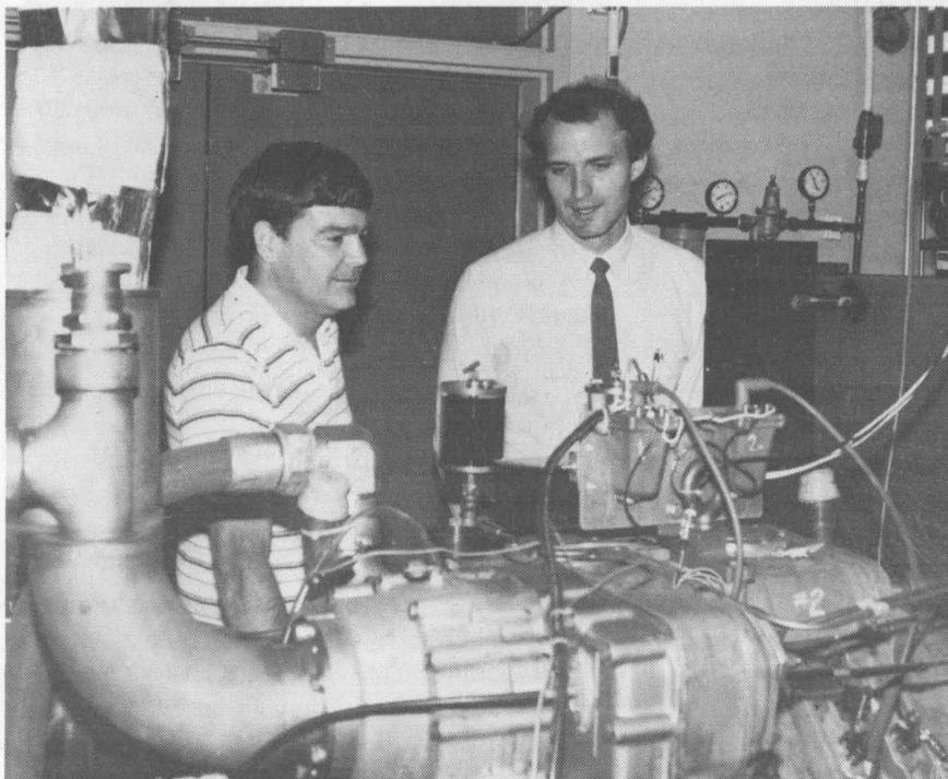
JOHN DEERE's prototype 750-horsepower rotary engine (foreground) got a workout while at CRF last year. Pete Witze (DMTS, 8362, left) and Philip Dimpelfeld (DOE Industrial Fellow from John Deere's Rotary Engine Division) ran the large Wankel-type rotary engine through its paces, measuring in-cylinder air velocities and turbulence to verify a John Deere multidimensional computer model.
