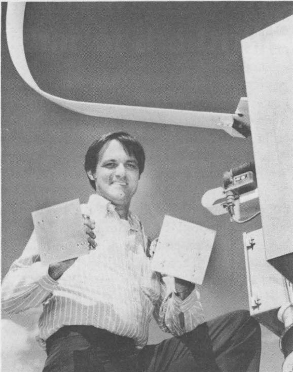
BILL SULLIVAN (now 2542) holds movable panels that automatically brake a vertical axis wind turbine (VAWT) in high winds. His patented "wind spoiler" moves on roller system from base of VAWT blade to equatorial center. Scale versions were proof-tested on Sandia's 5-metre VAWT.
