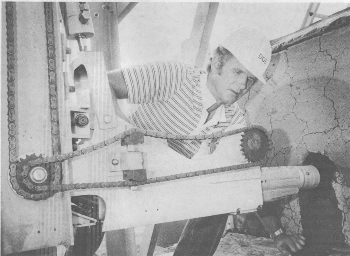
THIS DRILLING R&D relic being examined by Dave Shirey (5267) is the prototype cornering water-jet drill designed for use in coal mines. It died when funding for the Labs' fossil energy drilling program became a victim of budget cuts.
