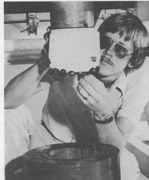
DURING THE HEIGHT of Sandia's drilling R&D activities, Dave Glowka (6252) often was found examining drag bits before testing in the Bit Hydraulics Facility. During testing, the rotating bit was situated inside a transparent plastic hole that simulated a borehole.
