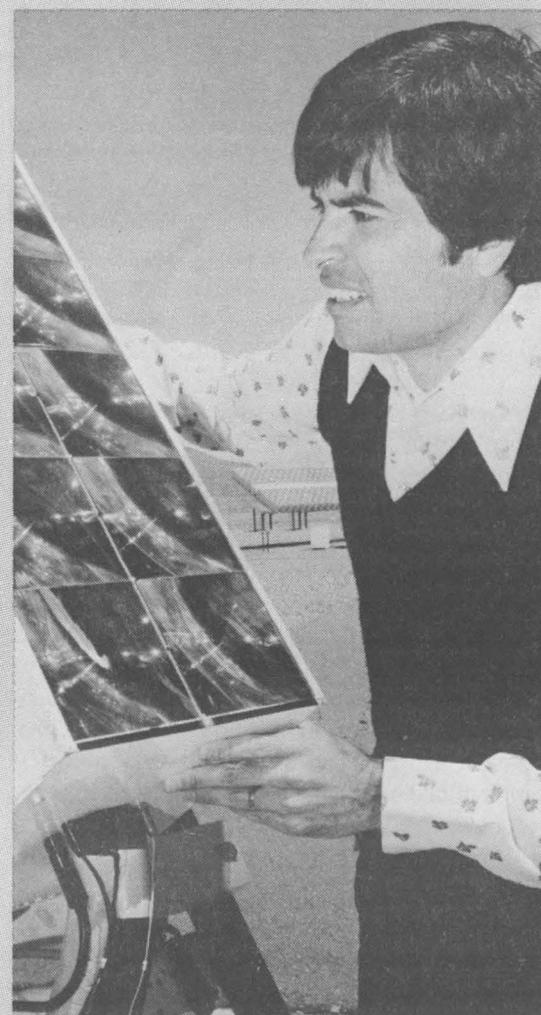
BACK IN 1984, Dan Arvizu (6224) was project leader for an experimental silicon solar cell module, which achieved a record-breaking — at that time — conversion rate of 17 percent.
