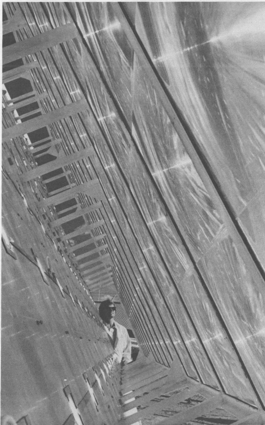
FIRST PV CONCENTRATOR ARRAY, designed and built by Sandia in the mid-70s, used 135 Fresnel lenses (right) to concentrate sunlight on an equal number of silicon solar cells (bright spots on left). The array's silicon cells achieved an unprecedented — for that era — 14 percent conversion rate, recalls Don Schueler (6220).
