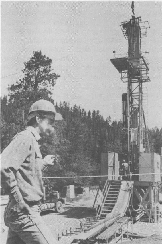
AS PETE LYSNE (6252) explains to a site visitor (out of camera range), the 50-ton drill rig sits 12 feet above grade (note rig wheels in large photo). The extra height permitted installation of main BOP (blow-out prevention) stack, a series of valves that can shut off the flow of fluids or gases to the surface whether or not a drill string is in the corehole.
