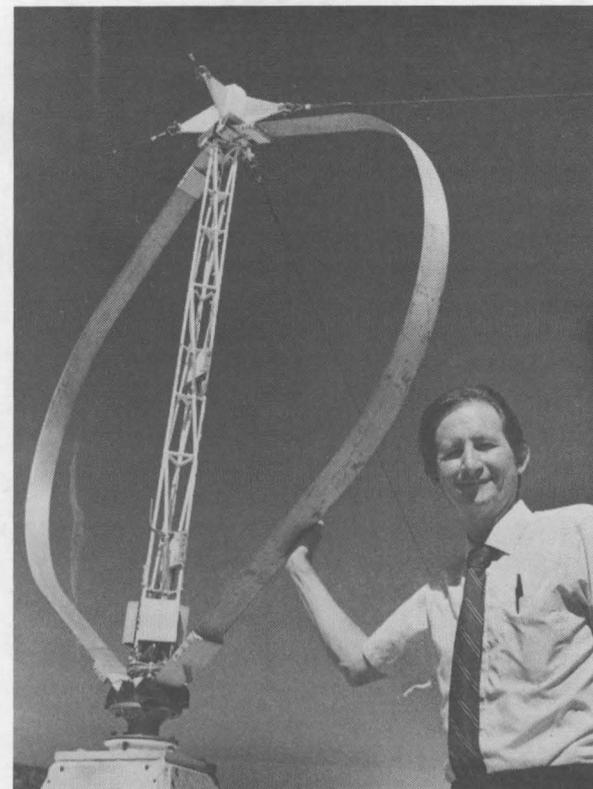
HERB SUTHERLAND (DMTS, 6225), recently inducted as a Fellow of ASME, is currently project leader for developing analytical techniques to determine the fatigue life of wind-turbine components. Behind him is Sandia's five-metre-diameter vertical-axis wind turbine.
