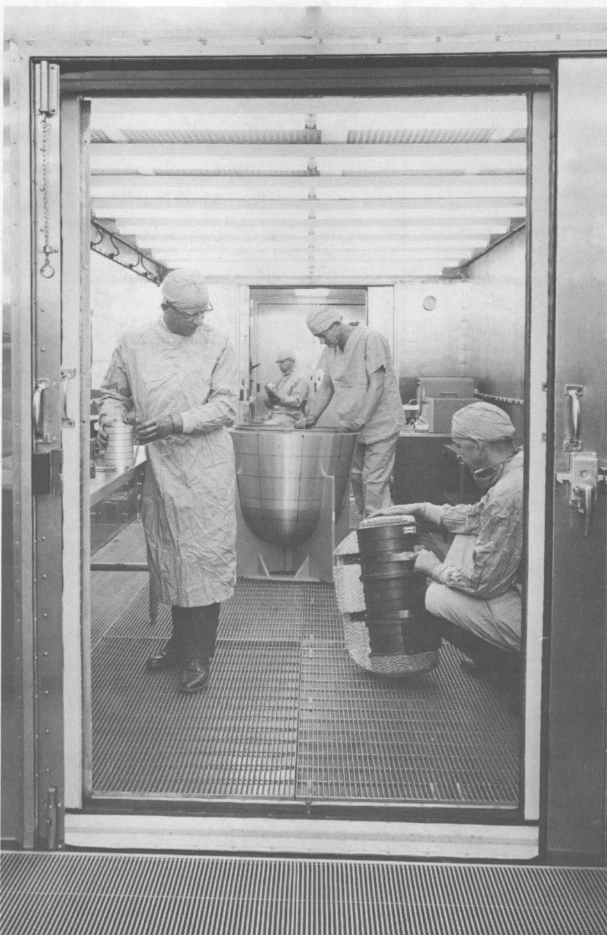
GORDON KING (left) with Sandia co-workers in the first vertical laminar flow clean room built at the Labs. The former Sandian led efforts in 1963 to establish a federal standard for defining clean air, an outgrowth of Sandia's invention of the laminar flow clean room. Federal Standard 209 quickly became the government and industry standard and has been disseminated and applied worldwide. Gordon later went on to work for Texas Instruments (TI), developing semiconductor facilities and designing clean room facilities. He's now retired from TI, but continues to do clean room design and fabrication consulting, working out of his small ranch in Eustace, Tex.
