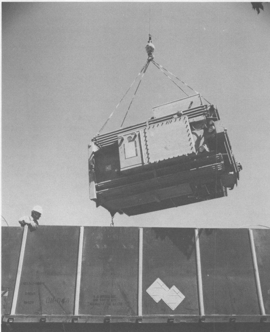
ONE FOR THE ROAD — Two giant transformers at Sandia, Livermore, weighing in at 12 and 14 tons, recently were removed from the premises. The transformers operated east of the steam plant for 30 years. When they were originally brought to Livermore by railcar, the event made front-page news as the largest delivery of utility equipment ever unloaded in town. The units have been trucked to Ohio, where a firm will dechlorinate the PCB oils and recycle them.
