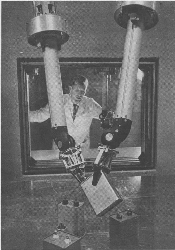
FORMER SANDIAN BILL BIRD operates the master-slave manipulators at the Sandia Engineering Reactor Facility (SERF) — Sandia's first reactor facility — in 1962. (Laskar photo)
