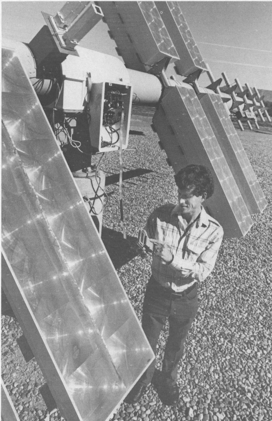
ALEX MAISH (6221) keys data into user-interface board to check the performance of the SolarTrak controller, an autonomous solar tracking system (in cubicle in center). The array tracks the sun in its path across the sky based on time readings and location rather than less-reliable sun sensor data. The system is being manufactured and marketed by three solar energy companies that have negotiated non-exclusive licensing agreements with Sandia. (Photo by Mark Poulsen, 3162)
