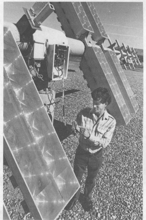
ALEX MAISH (6224) keys data into a user interface board to check the performance of the Solar-Trak controller, an autonomous solar tracking system (in cubicle in center). The array tracks the sun in its path across the sky based on time readings and location rather than less reliable sun sensor data. The system is being manufactured and marketed by three solar energy companies that have negotiated non-exclusive licensing agreements with Sandia.
