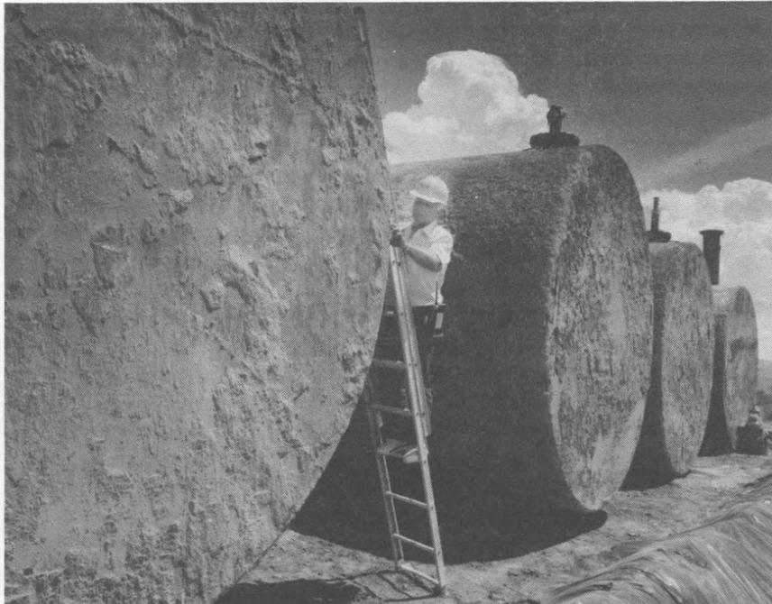
UNDERGROUND STORAGE TANKS, removed this summer, are inspected by Art Rodriguez (7721). The locations where a number of aging underground tanks were removed are on Sandia's list of sites to be assessed and dealt with as part of the environmental restoration program.
