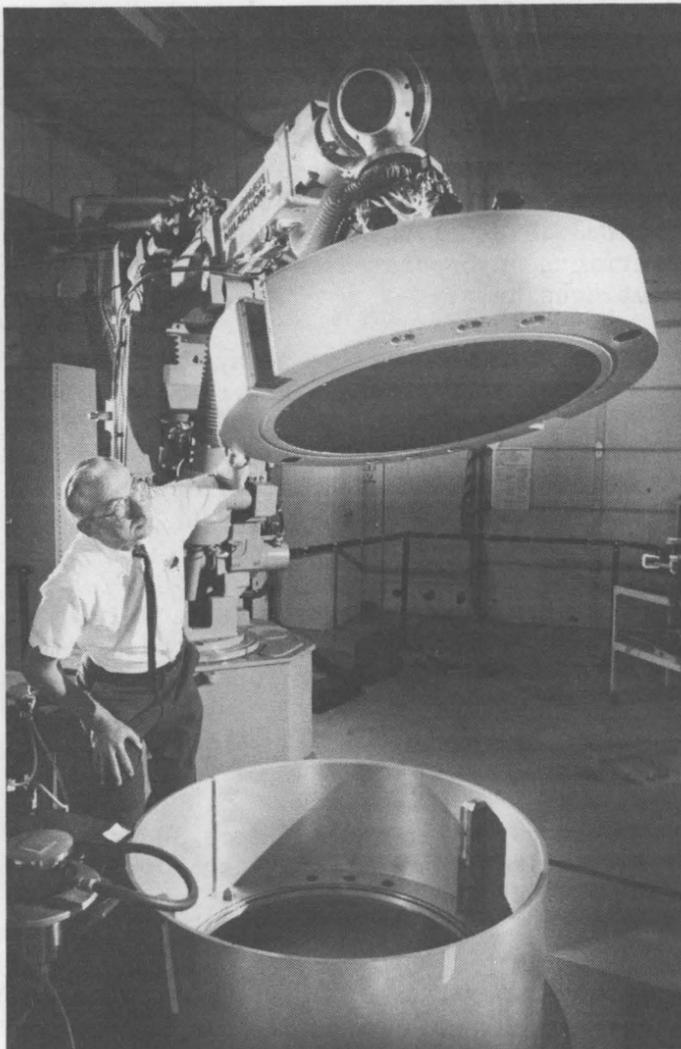
EXTENDED FAMILY of "smart" robots is helping automate a variety of DOE operations. In Sandia's robot lab, researchers are developing a system that inspects lids on transport casks for high-level radioactive waste. Ben Petterson (1416) is seen checking the underside of a full-scale model of such a cask lid at Sandia's inspection station. (See "Automated Handling Techniques Reduce Waste, Hazards" on page five.) (Photo by Randy Montoya, 3162)
