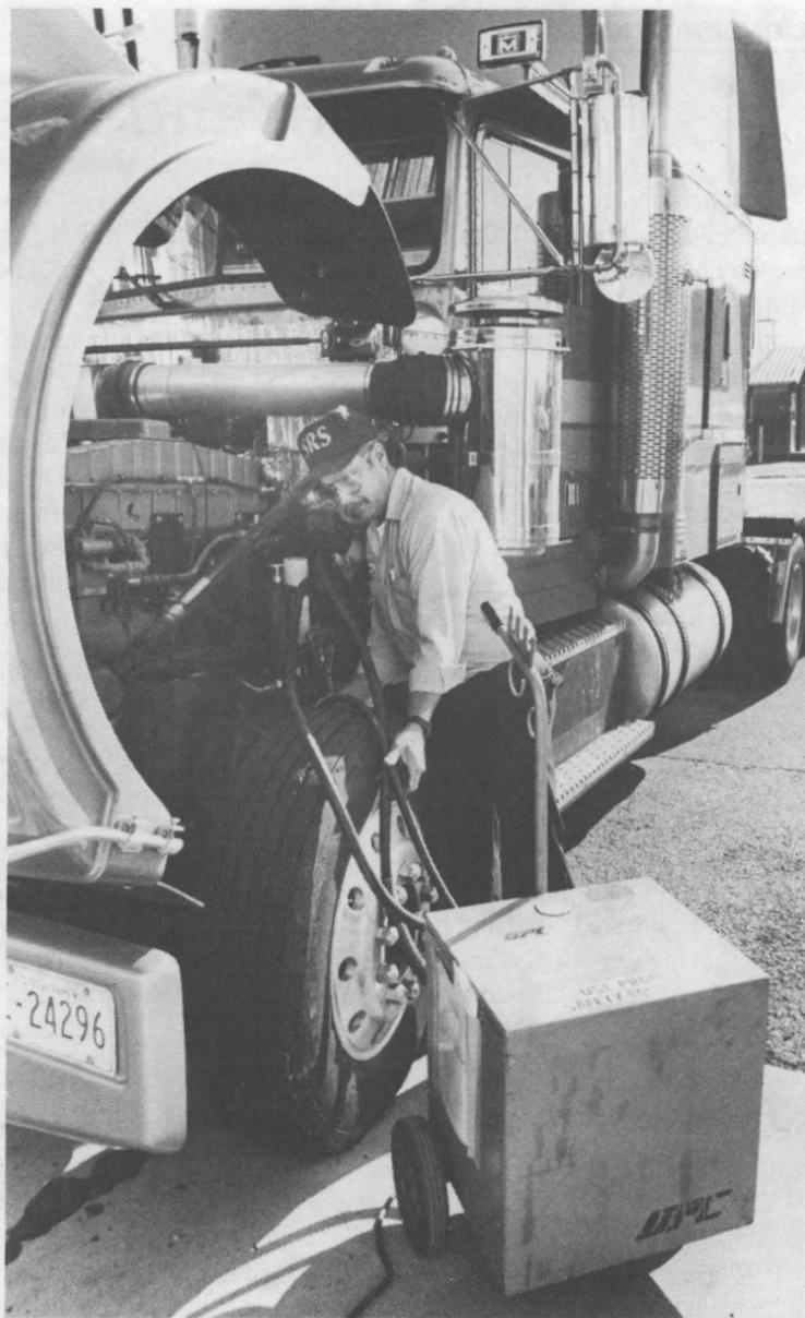
**BLENDED THE OIL** — Fred Raether (3423) connects a blender that takes oil from the crankcase of this DOE tractor, filters it, and mixes it with the tractor's diesel fuel. This use of motor oil, approved by the engine manufacturer and certified by the EPA, saves the cost and the environmental impact of disposing of it as hazardous waste after an oil change.
