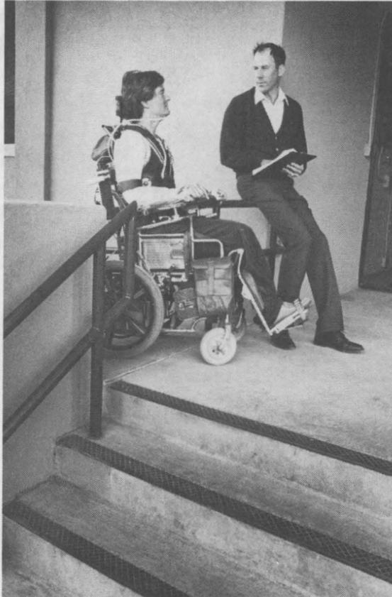
AT THE TOP of a new wheelchair ramp in front of Bldg. 836, Blase Gaude (5021, left) and Wayne Burton (7845) discuss recent facilities work that has improved accessibility to the building for people with disabilities. A sensor above the ramp triggers automatic foyer doors, and a button inside the building opens the doors as well. Before the new ramp was installed, the steps in the foreground were major obstacles for employees with disabilities.
