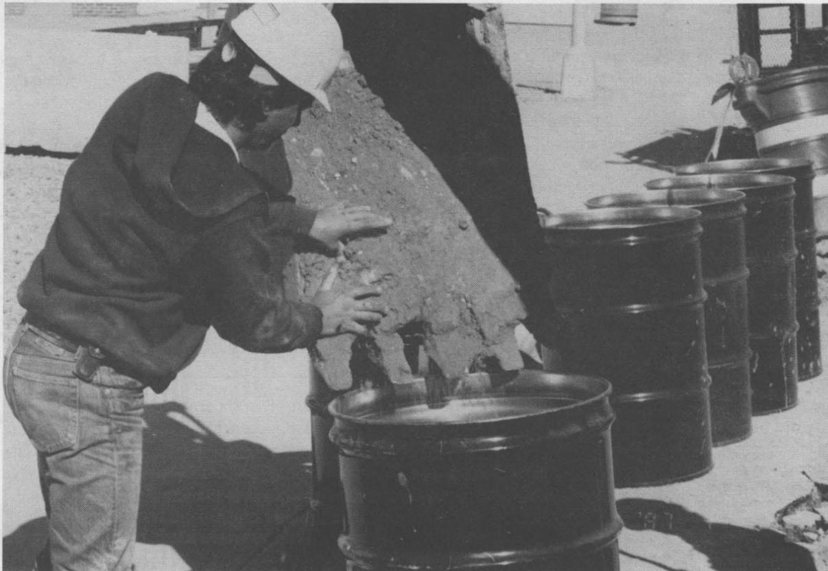
**BOLTS AND DIRT** exhumed from a construction trench inside Tech Area 1 are guided into 55-gal. drums by a member of a contract construction crew. Because some of the counterfeit bolts were plated with cadmium, the bolts were sifted from the dirt and sent to a hazardous waste disposal facility in Louisiana.
